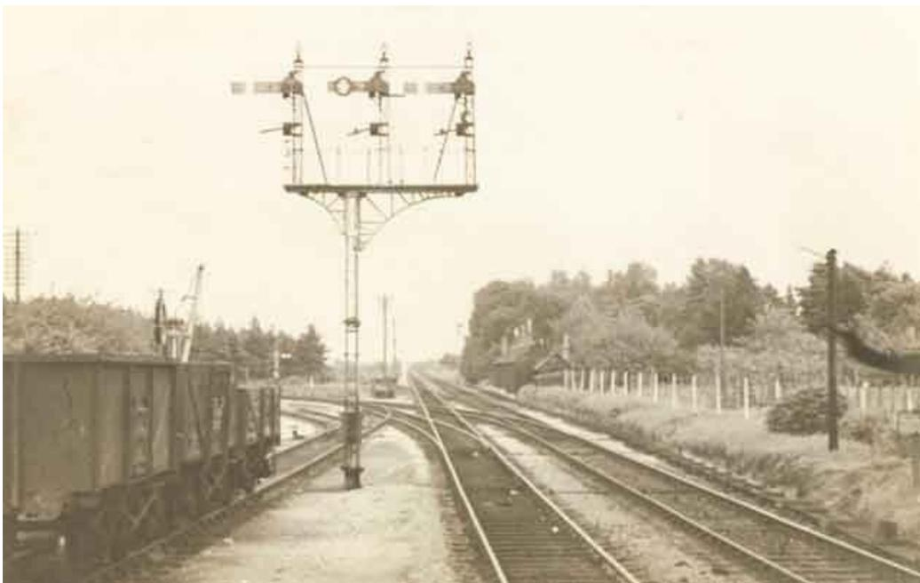
This view (above) shows the junction more clearly together with the iconic junction signals. The middle semaphore arm, with the circle attached, controlled traffic entering the MOD fuel depot sidings network. On the right of the tracks in the middle-distance can be seen the long line of single-storey ‘railway cottages’, dating from the middle part of the 19<sup>th</sup> century.
